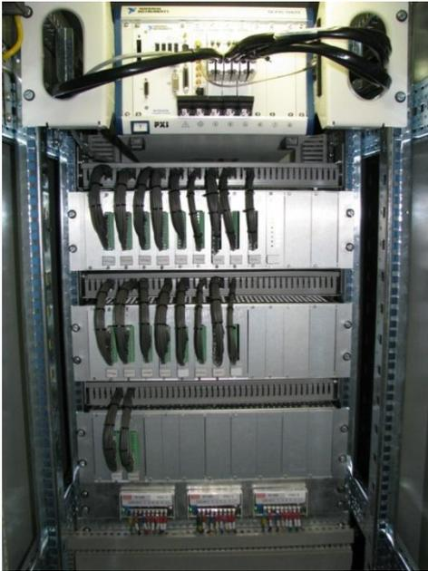
Fig. 4. 11kV substation monitoring equipment.
