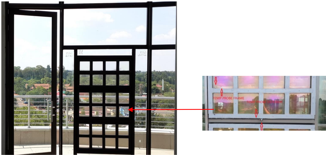
Figure 8. Installation of Panels and Monitoring Sensors
